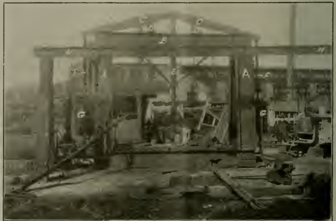
PRESS FOR STRAIGHTENING BENT AND DISTORTED MATERIAL, RECLAMATION PLANT, VIRGINIAN RAILROAD.
